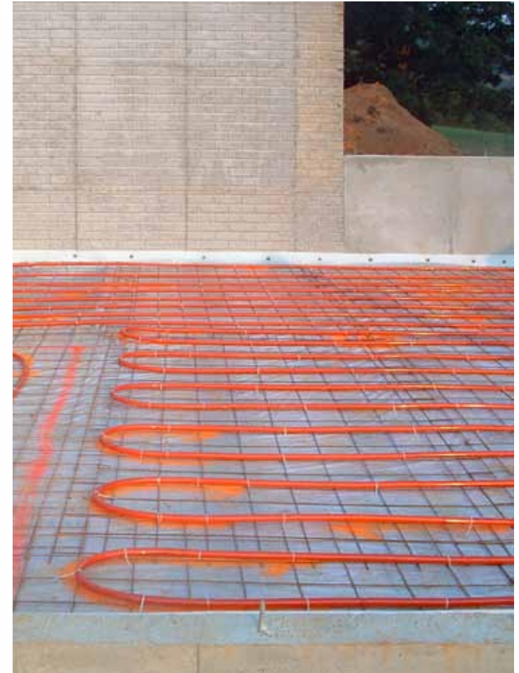
As a prototype for sustainable dwelling, the house extracts energy from the ground with a geothermal heat pump connected to a radiant slab and air handler. The roof was designed and has been prepared for both thermal and photovoltaic panels on the south-facing leaf.
